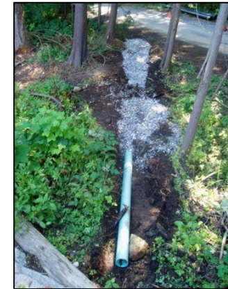
Above - Drainage outlet retrofitted from #4551 through park to Clovelly:
