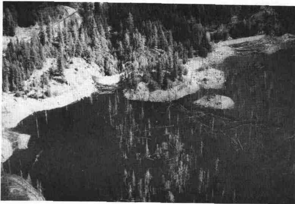
Photo 28 THIRSK RESERVOIR - Looking East (Sept. 12, 1973) Trout Creek System
