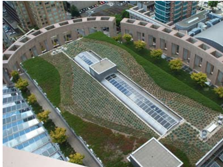
Vancouver Public Library green roof.
