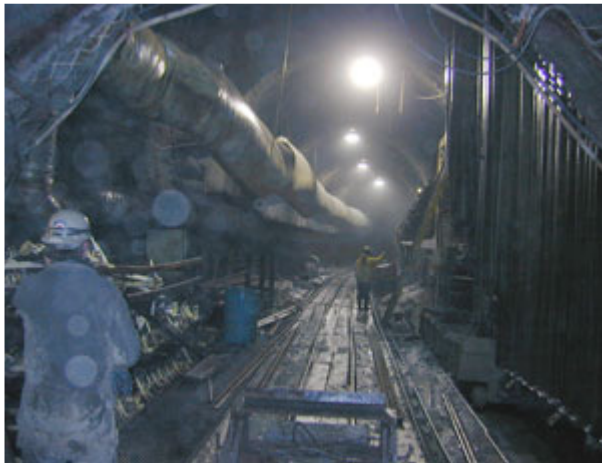
Photo: Courtesy of Northeast Ohio Regional Sewer District
