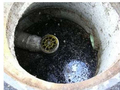
Hanging trap installed in a sedimentation manhole
