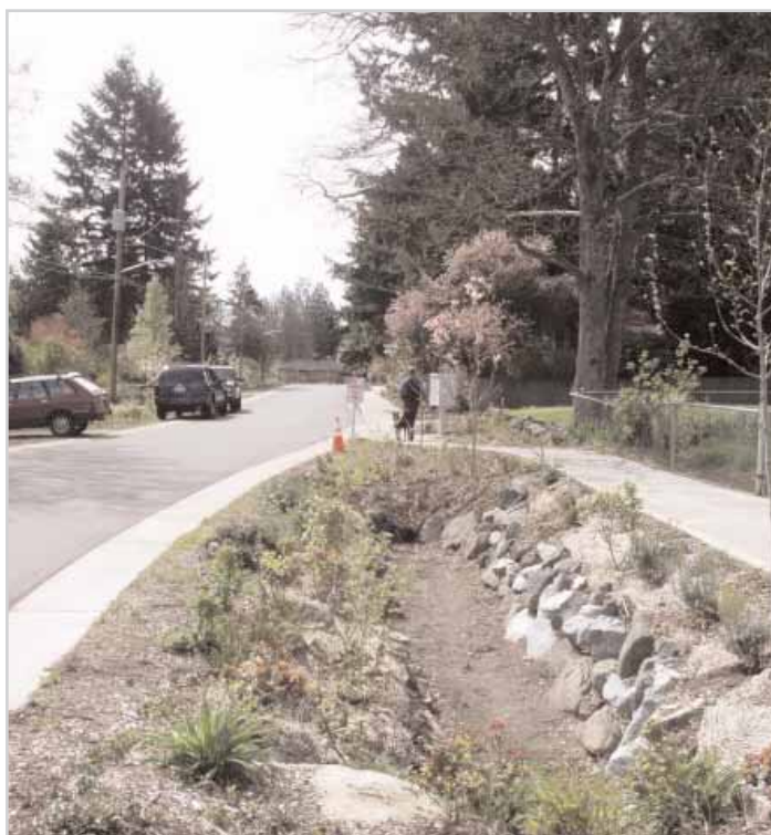
A retrofitted residential street in Seattle, WA, includes trenches and no curbs.
