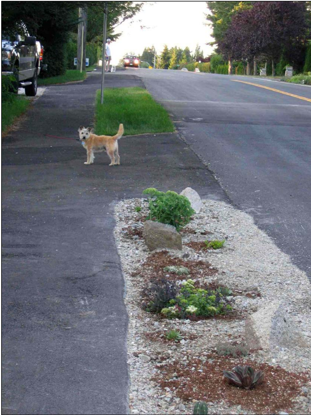
At-grade asphalt sidewalk; typical grass swale in background and resident's landscaping additions in foreground
