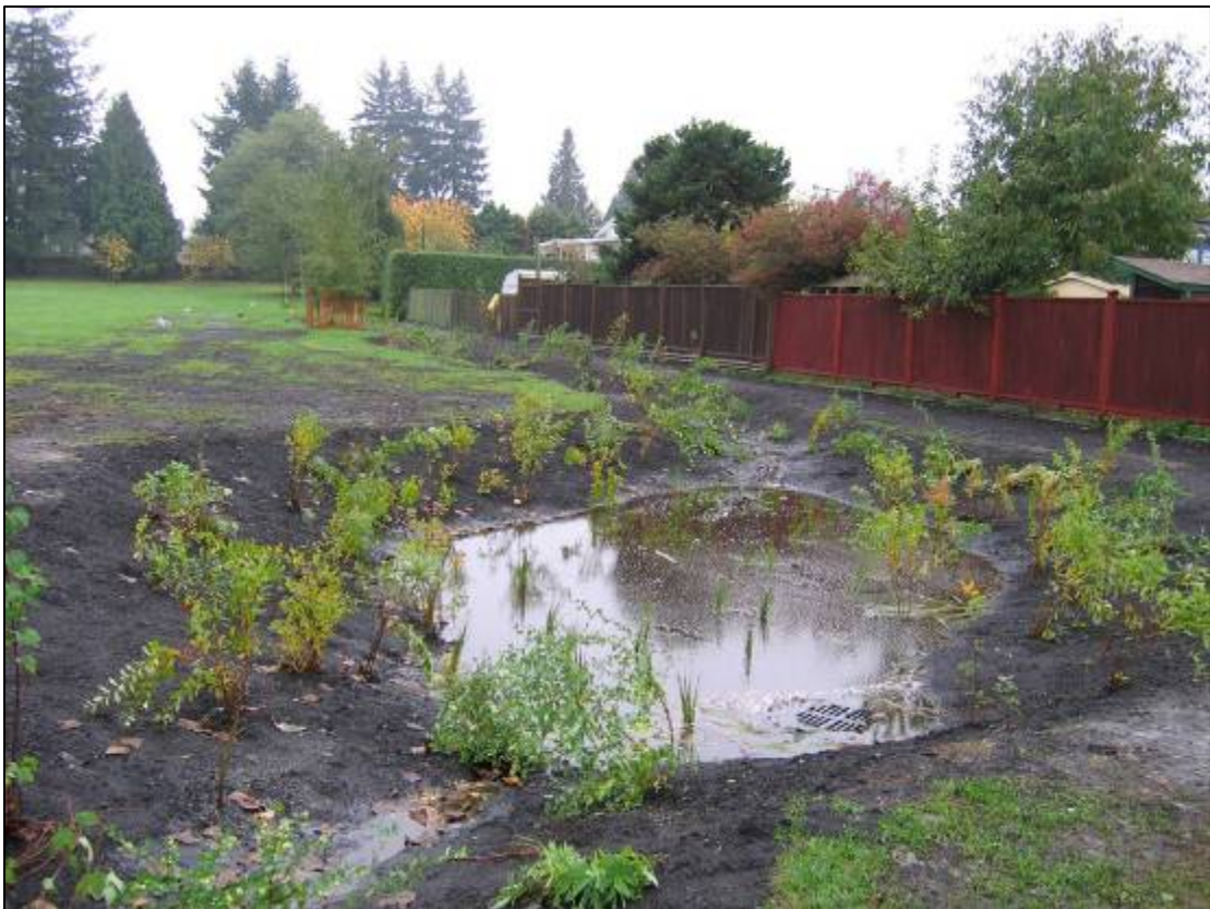
Swales flowing into rain garden pond (October 2005)
