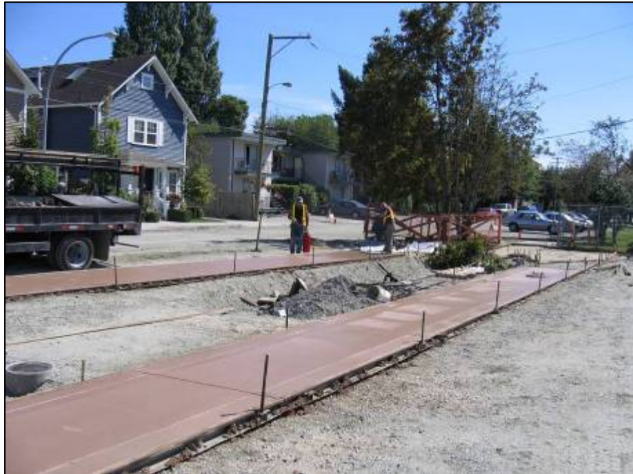
Sidewalk around planting area under construction
