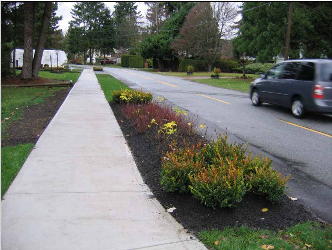
Swale plantings (November 2007)
