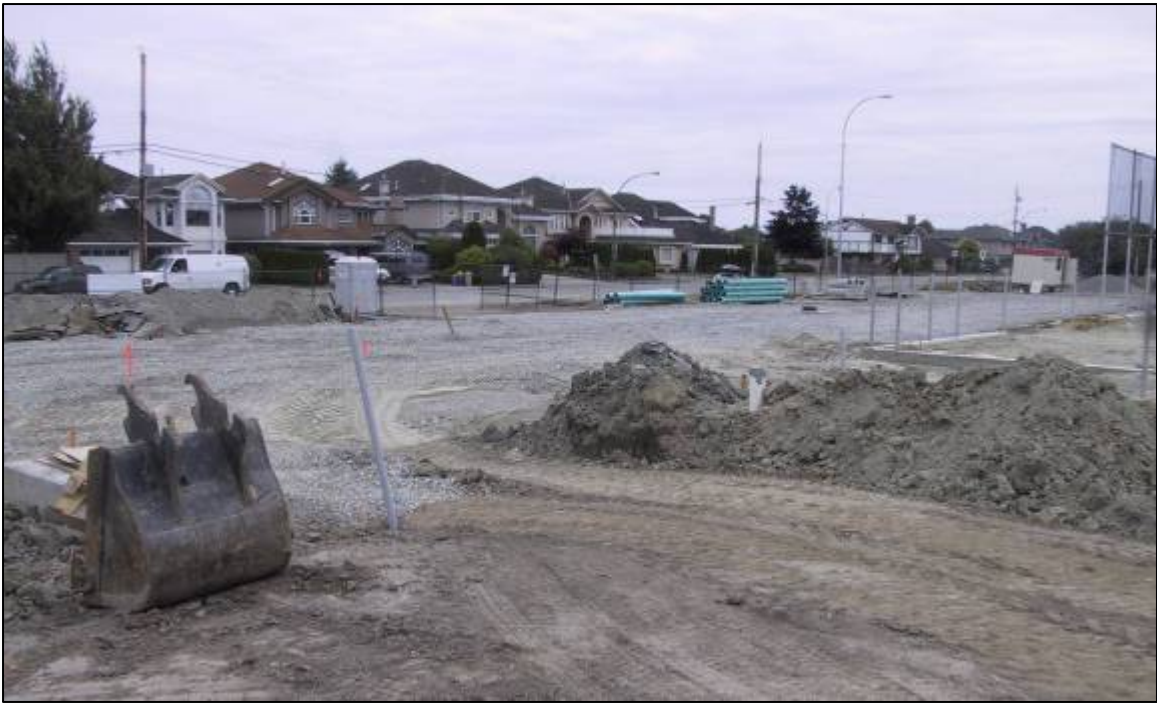
Parking lot under construction
