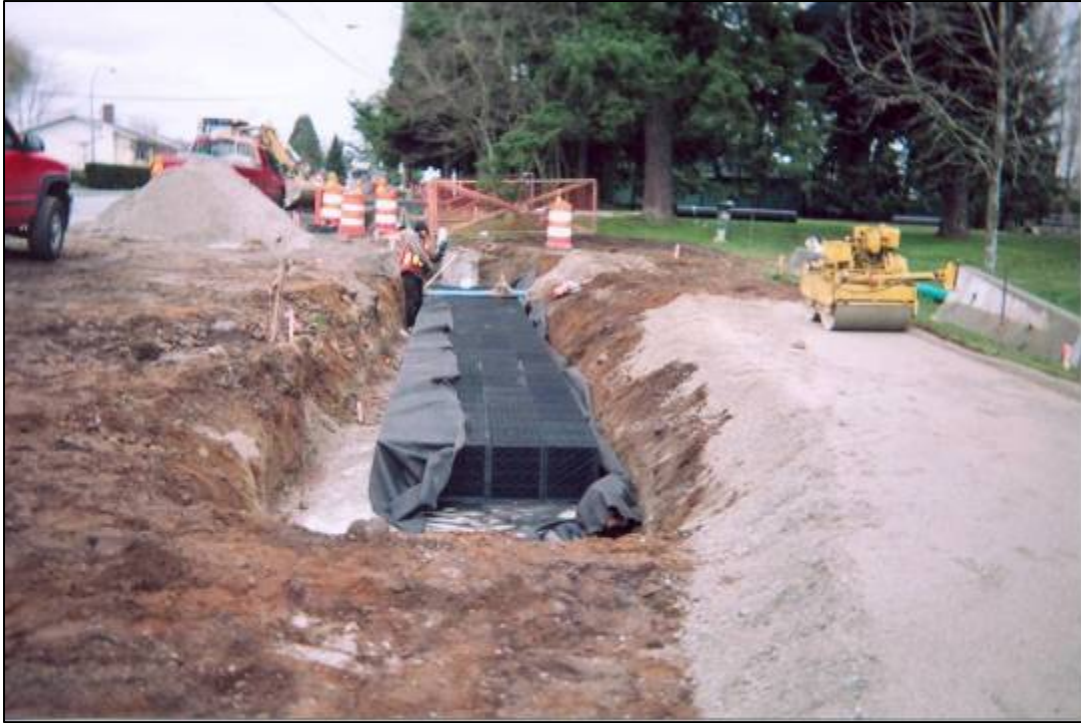
Construction of underground infiltration gallery
