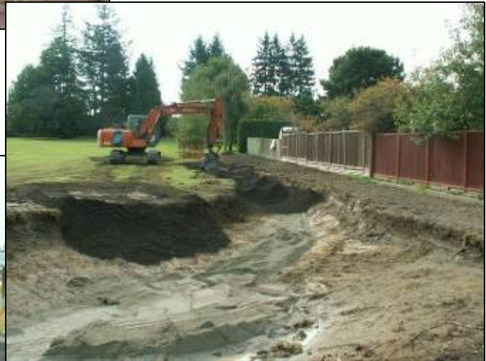
Swale under construction; installation of sand and topsoil
