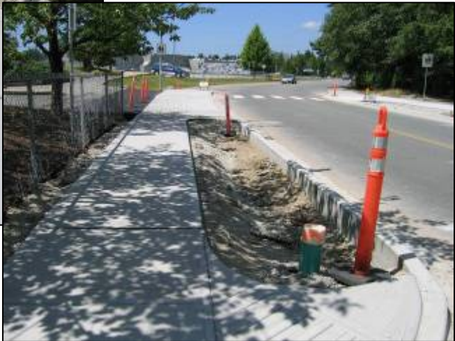
South side during construction
