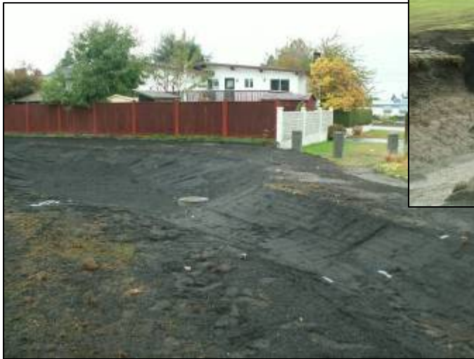
Final grading of topsoil complete
