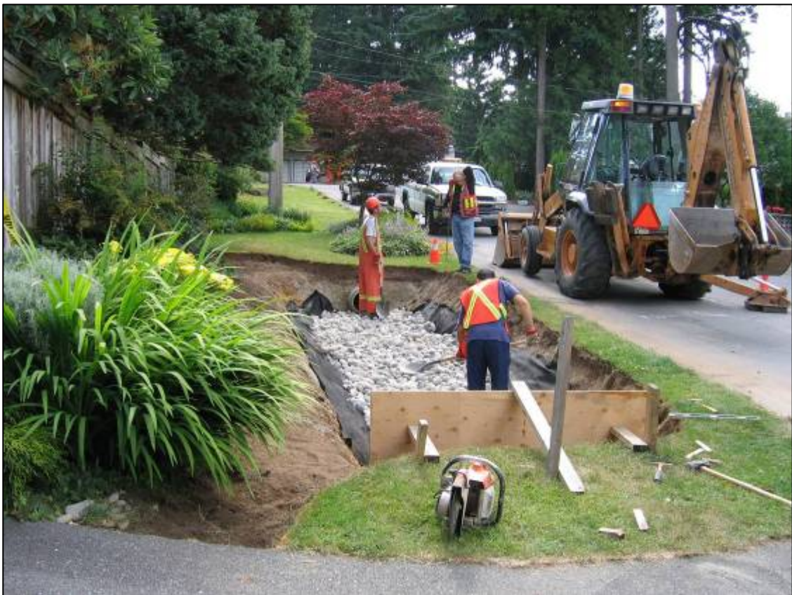
During construction (June 2006); installing river rock over wrapped drain rock
