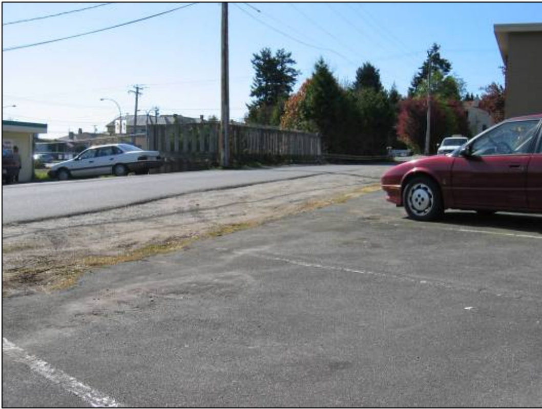
BMP area prior to construction
