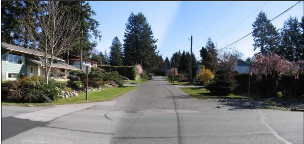
Pre-construction condition (spring 2006)
