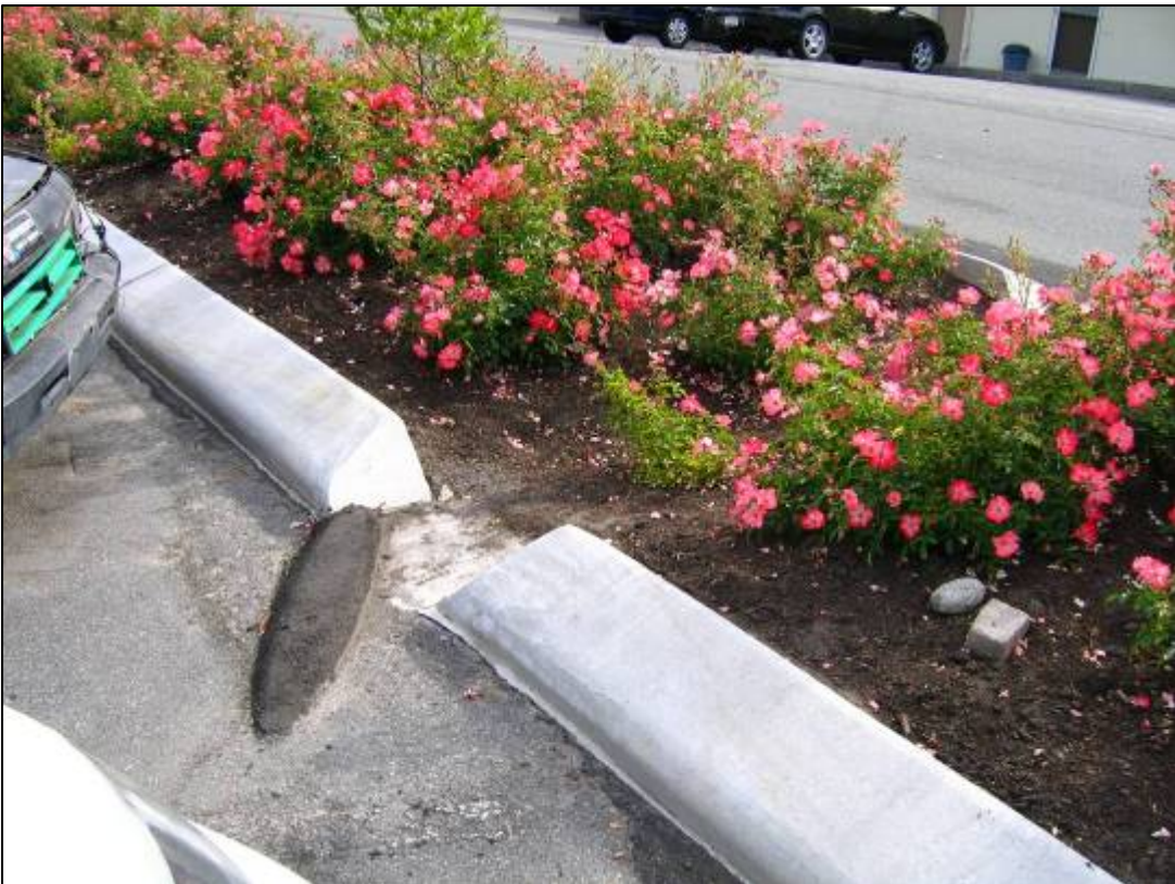
Asphalt diverter for directing drainage into planter
