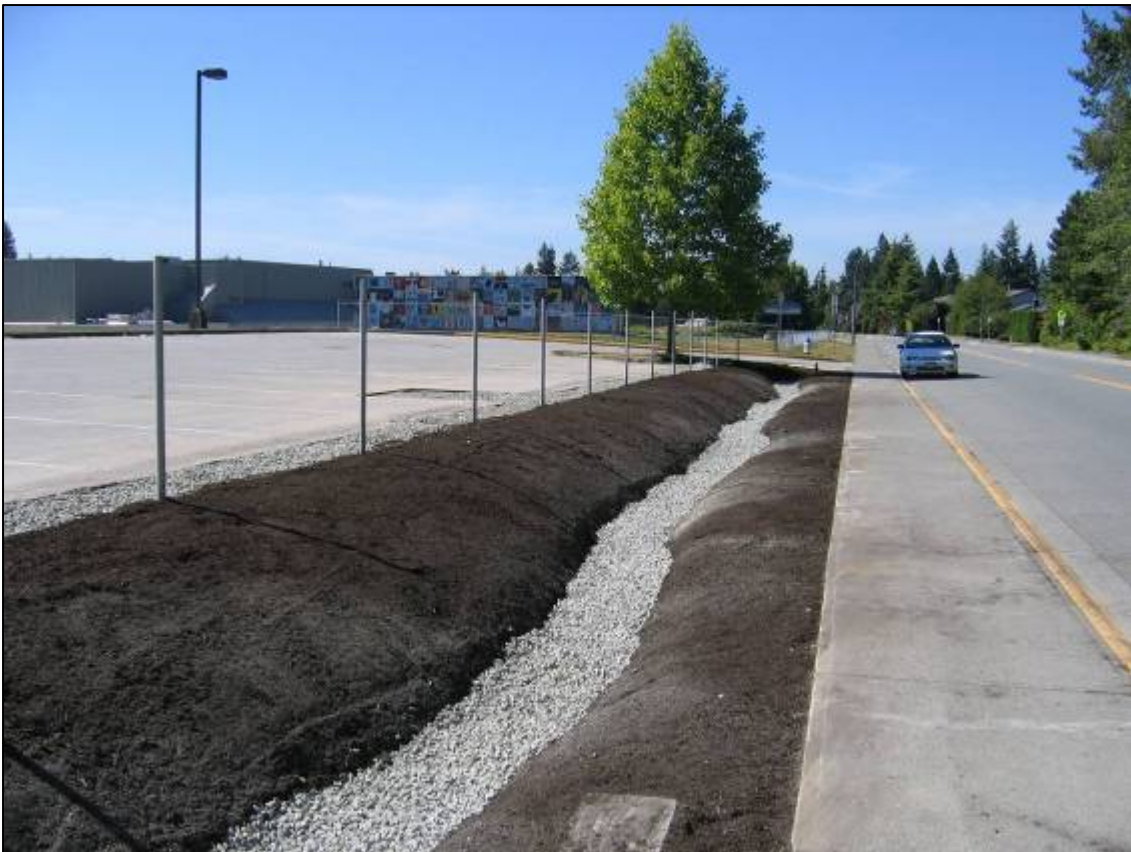
Swale completed (August 2006)
