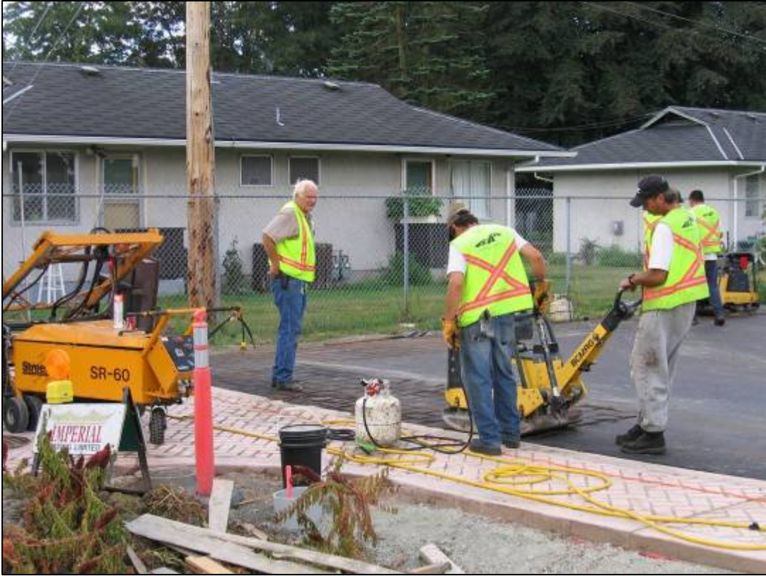
Stamped asphalt parking lot under construction
