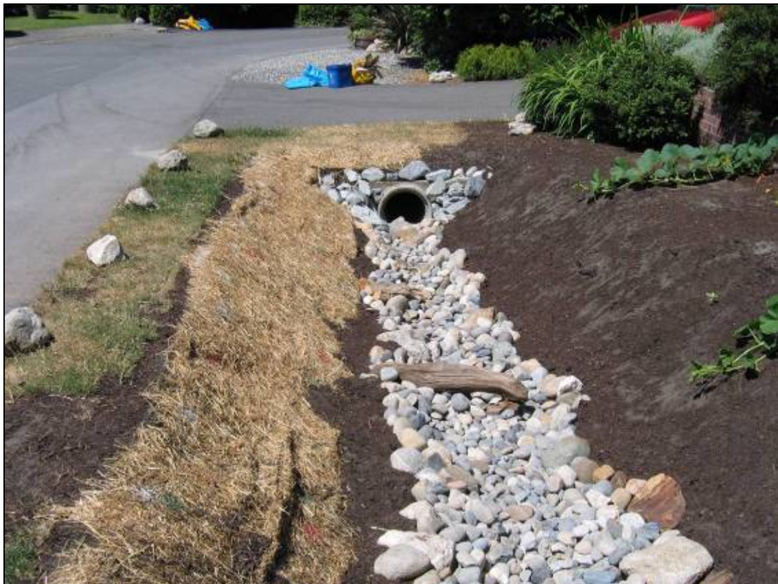
After resident added driftwood and boulders (July 2006)
