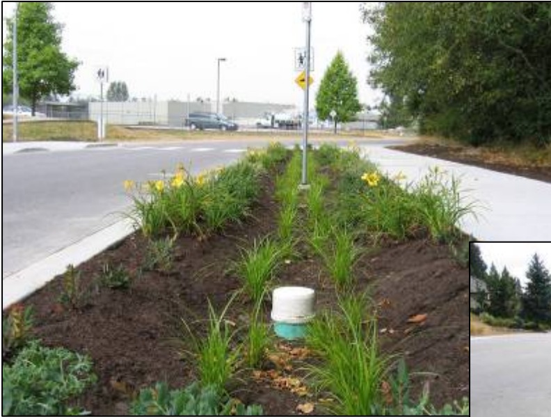
North side after planting; overflow grate still to be installed on pipe in foreground
