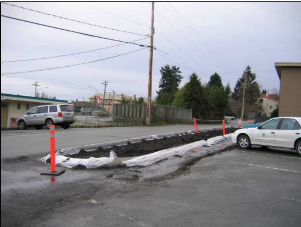
After construction (January 2006)
