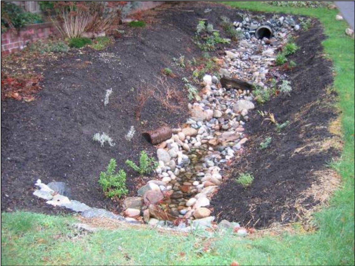
During heavy rainfall event (November 2006)
