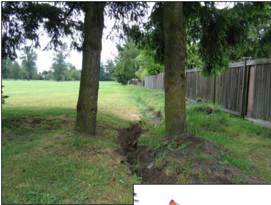
Temporary trench (summer 2005)
