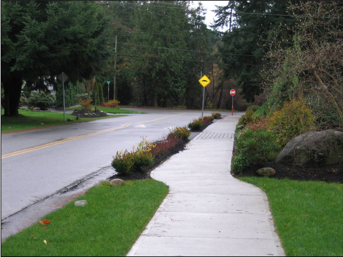
Low shrubs planted in narrow section between road and at-grade sidewalk discourage parking on sidewalk and separate traffic from pedestrians (November 2006)
