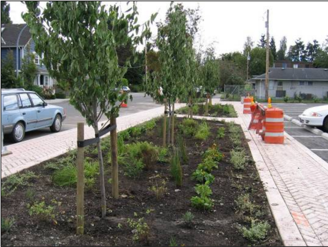
Planting beds for stormwater collection (east side)
