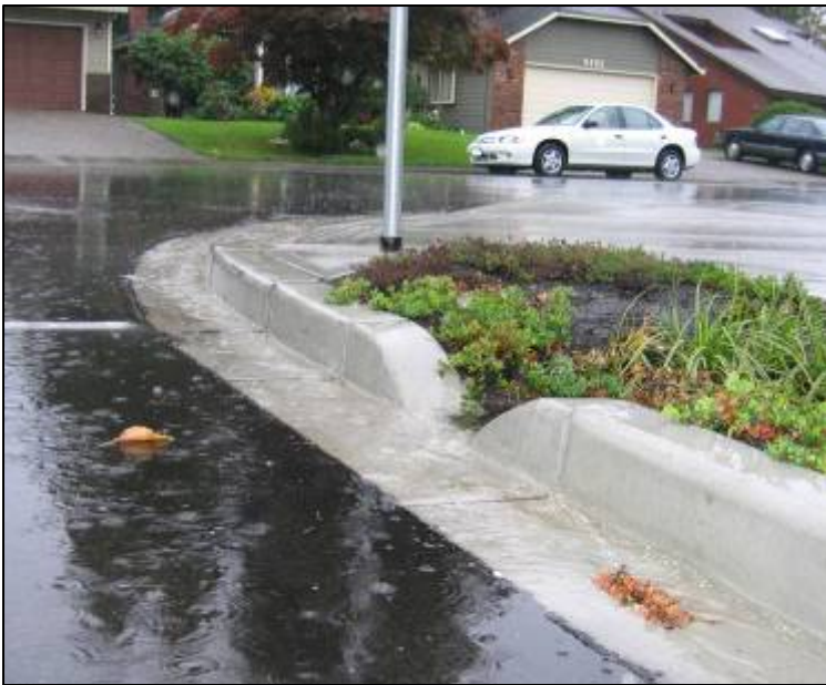
BMP during heavy rainfall event; water not absorbed as desired due to high soil levels in planted area
