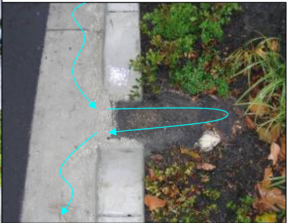
Extent of runoff into swale
