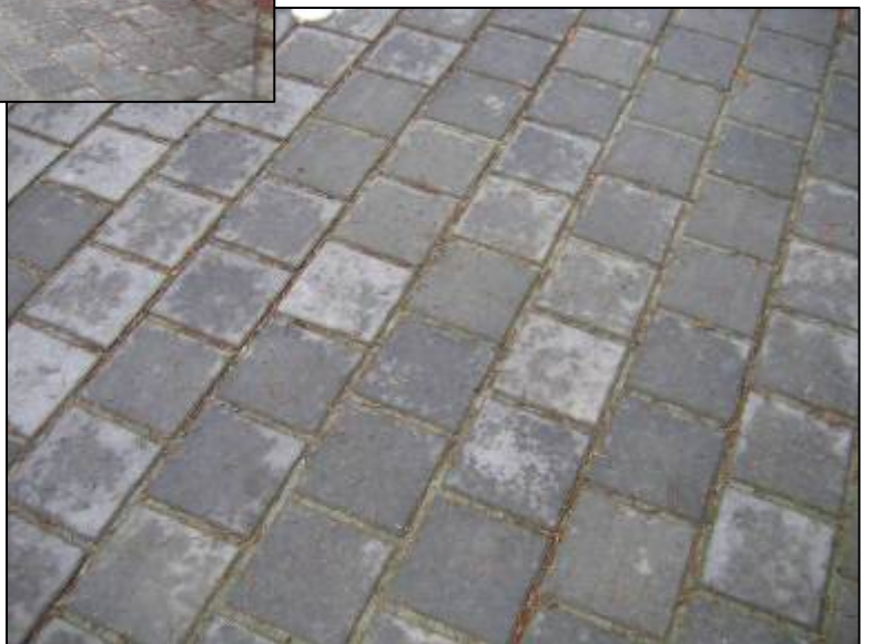
SF-Rima 200mm x 200mm x 80mm permeable pavers
