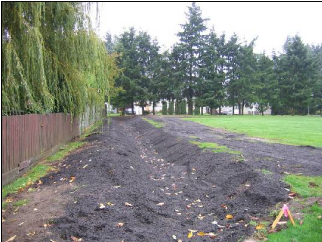
Completed swale with berm on fence side (October 2005)
