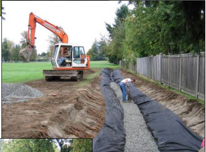
Installation of drain rock
