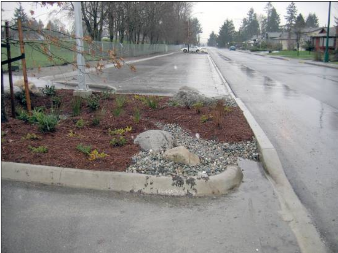
After construction (January 2007). Rain gardens collect and infiltrate water from paved parking areas.
