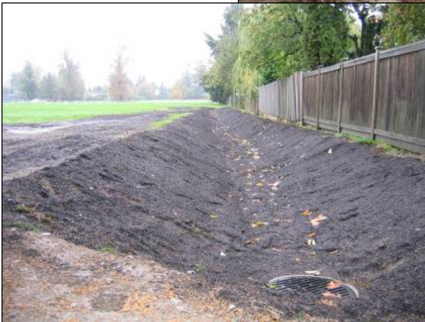
Completed swale (October 2005)
