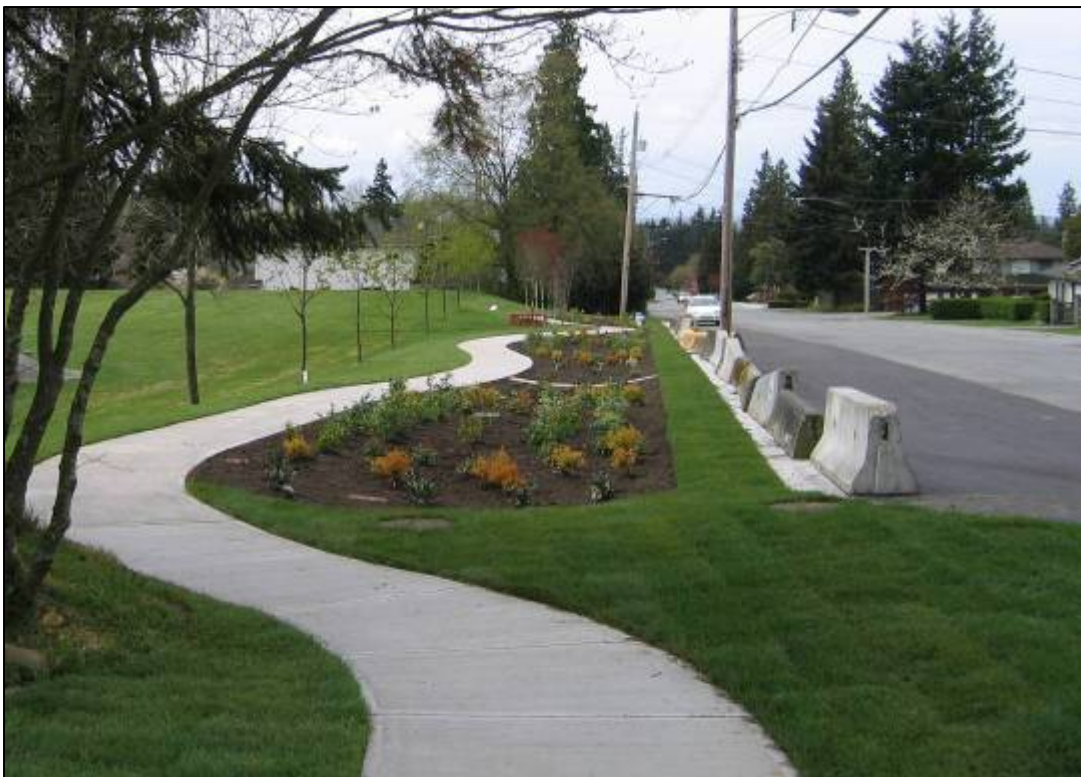
After construction and planting (April 2006) – barriers were later removed
