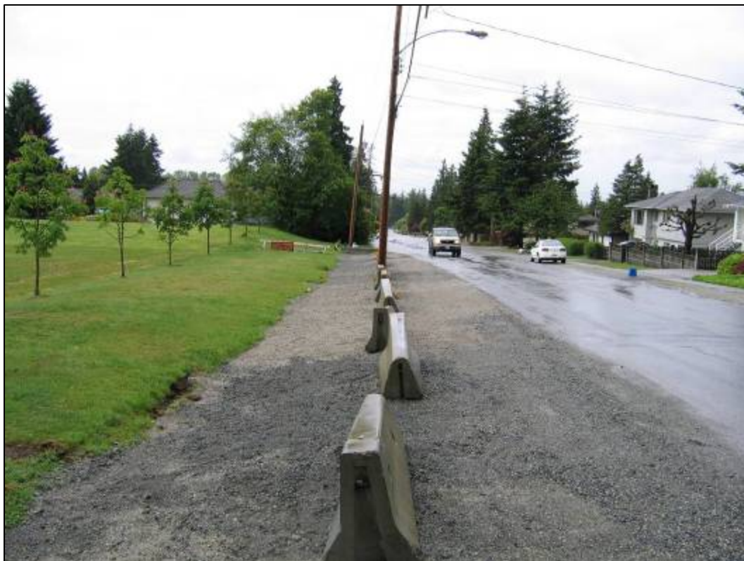
Pre-construction site conditions (after ditch infill)
