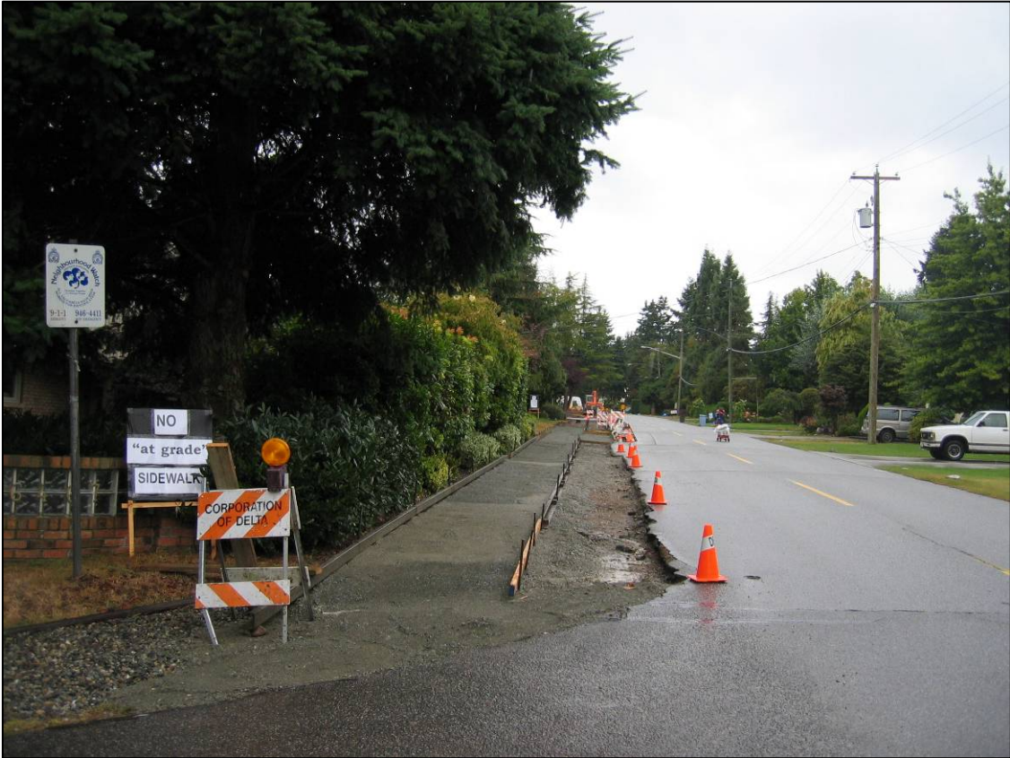
Knight Drive at-grade sidewalk under construction (November 2006)
