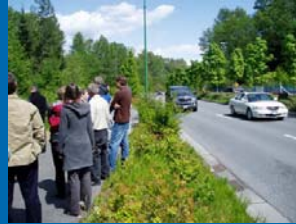
An Arterial Highway
