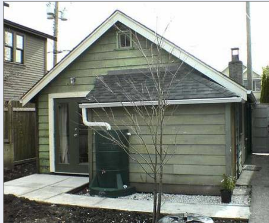
Rain barrel at infill dwelling, Vancouver
