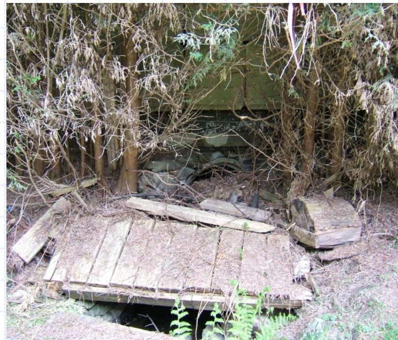
Photo 2, Culvert Inlet at 142 nd Street
