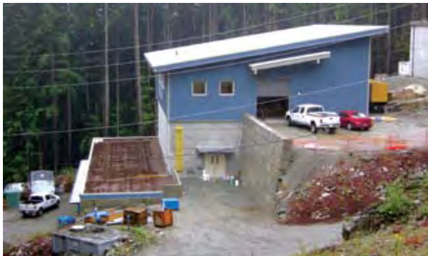
Eagle Lake Membrane Filtration Facility. A tiered vertical structure was designed to follow natural rock bluffs at the site.
