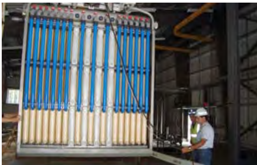
Membrane module being installed.
