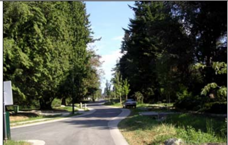
Minimum impact Street. No curbs or gutters, or drainage pipes. All surface runoff is infiltrated
