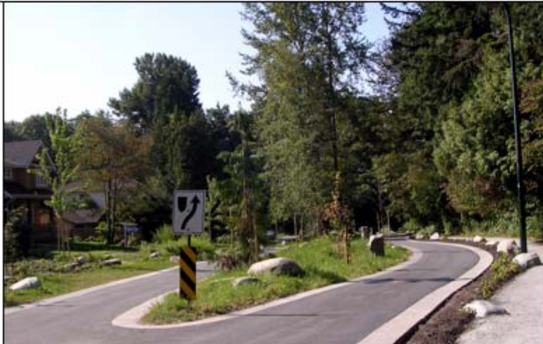
Minimum impact Street. No curbs or gutters, or drainage pipes. All surface runoff is infiltrated
