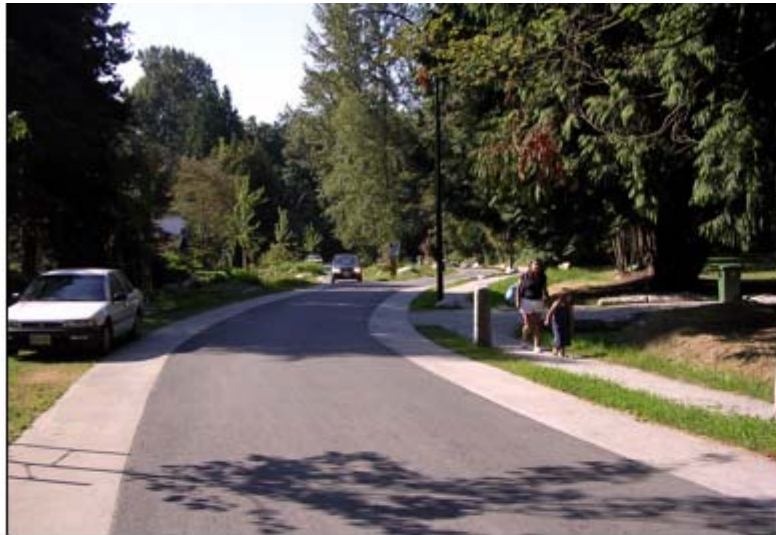
Minimum impact Street. No curbs or gutters, or drainage pipes. All surface runoff is infiltrated
