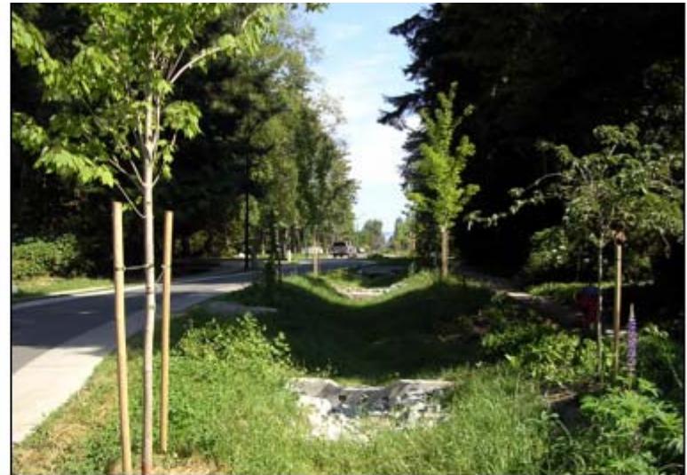
Minimum impact Street. No curbs or gutters, or drainage pipes. All surface runoff is infiltrated
