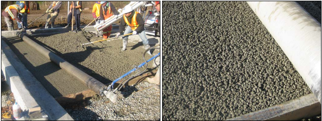
Fig. 4.2 – Spreading, strike-off and compaction of the pervious concrete.
