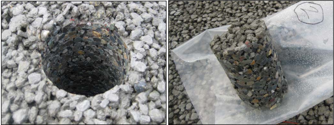
Fig. 5.2 – Cores were extracted to inspect compaction through pavement depth.
