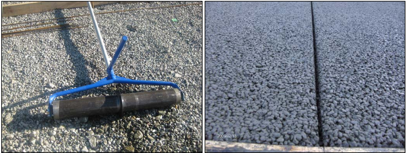
Fig. 4.3 – (c) Jointing tool and finished joint
