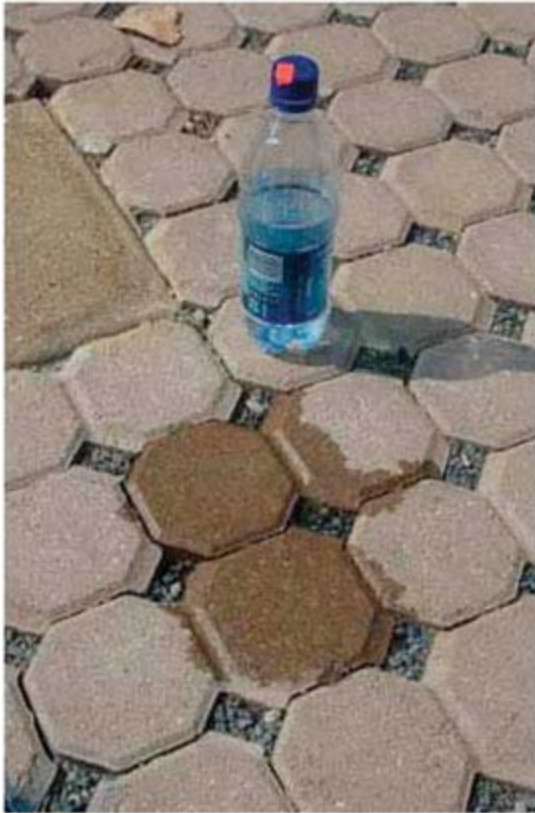
Photo: Bruce K. Ferguson Permeable pavers in Minnesota correctly installed with highly permeable single-sized aggregate in the joints
