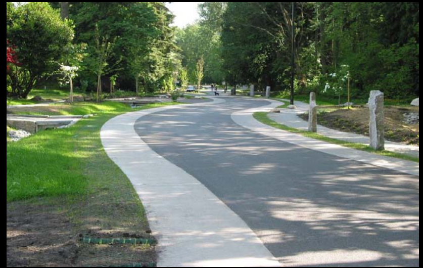
After reconstruction – green and inviting!
